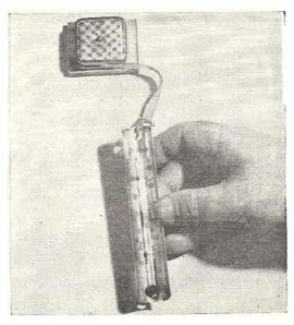
A spring measuring tape fastened to the wall over the developing bench makes thermometer handy, as shown above. When not in use, the tape readily winds up.
