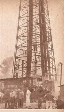
With the "fogger" in operation, men dare to come right up to the well. Fumes are blown away by the current of air, and fog makes ignition virtually impossible, enabling cappers to go ahead with their vital work.
