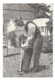
A scientific lawn aerator or sod spiker loosens the sod from underneath and cultivates the soil, thus making the lawn porous without tearing or disturbing the grass.
