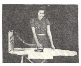
This tightly coiled ironing cord is always out of the way. When fully stretched the cord measures a little over seven feet and when released coils into a compact unit eight inches long. It is rubber covered and retains its coiled position for many years.
