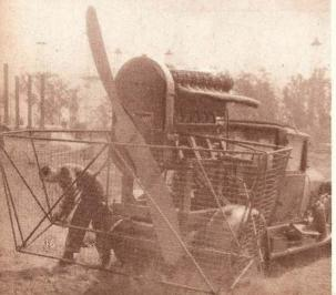
The first point of attack in capping a rampaging gas well is to produce an artificial fog. The "fogger" at the left reduces the danger of sudden oxidation.
