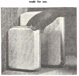
Coarse corrugated board, waterproofed with paraffine may be used for draining trays as shown above. Place the cardboard close to the wall to partly support trays.
