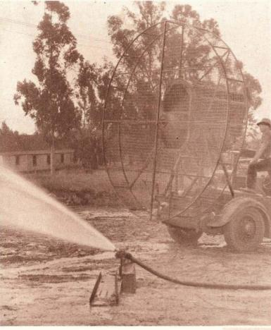
The "fogger" in action. With the prop going full blast, a two-inch hose runs a high pressure stream in front of the wind current, resulting in a fog.
