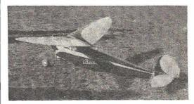
Buster Meeteer of the university city of Madison, Wis, sends in a picture of his gasoline model airplane which he named the Buster after himself. For his work he gets an award of \$3. The plane is 53 ½ inches in length and has a wing span of six feet. The power plant is a 1/5 horsepower engine. The Buster has had 26 successful flights, its builder reports.
