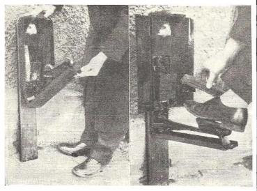
This compact shoe shining kit for the home unfolds quickly to permit immediate use. The bottom is hinged so that, when the cover is lowered, the sides project outward. The inside cover contains the foot rest.
