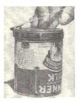
A simple device opens and reseals milk cans. A girdle with a bar hinged to it encircles the top of the can. Two spikes on the bar punch outlet holes in the can. Spikes also plug up the holes when the bar is held down by a friction clamp.
